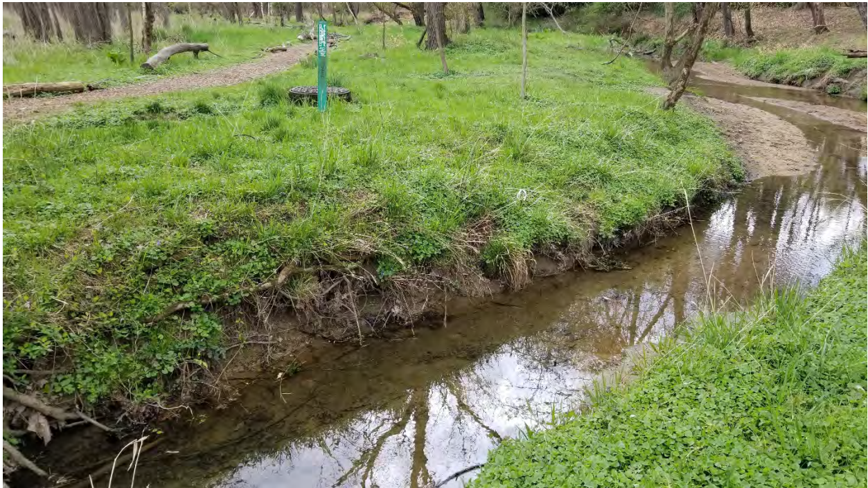
Photo 13: Walking path and sewer manhole adjacent to Plumtree Branch. Many utilities are present in the project area.
