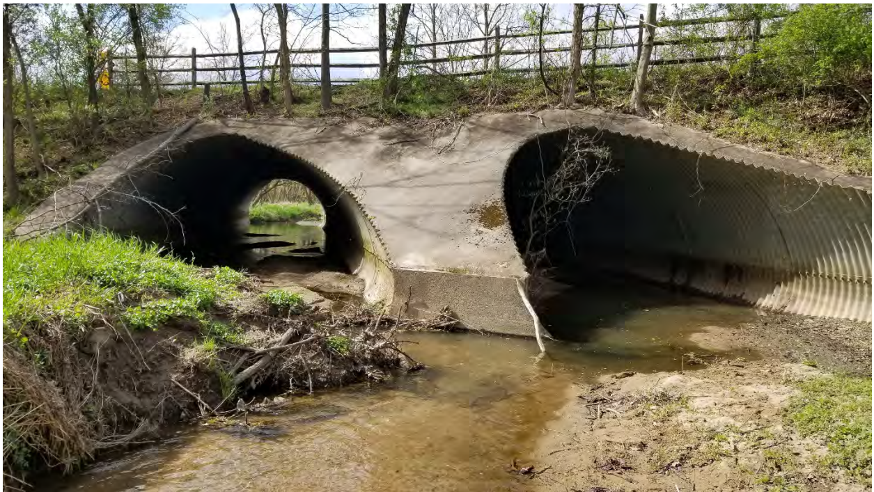
Photo 15: Culvert under Columbia Road.
