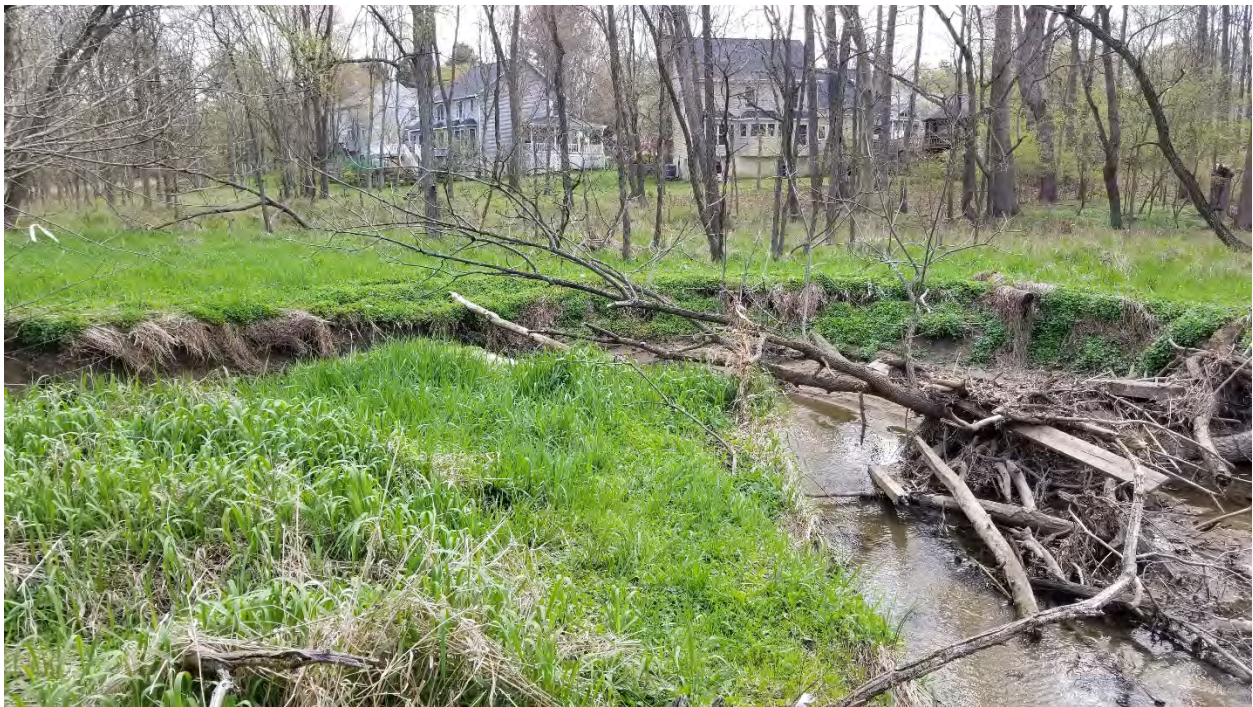
Photo 11: Vertical bank erosion on the outside of the meander.
