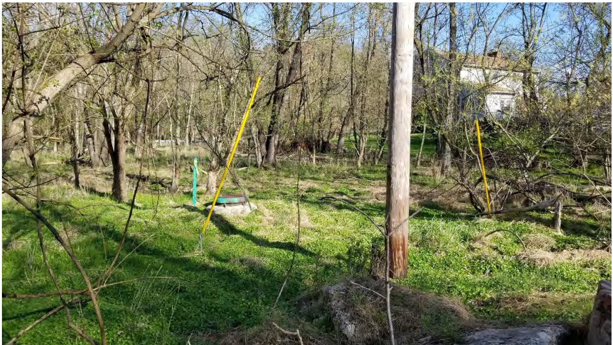
Photo 4: Manhole and utility pole on the right bank of the unnamed tributary. Many utilities are present in the project area.
