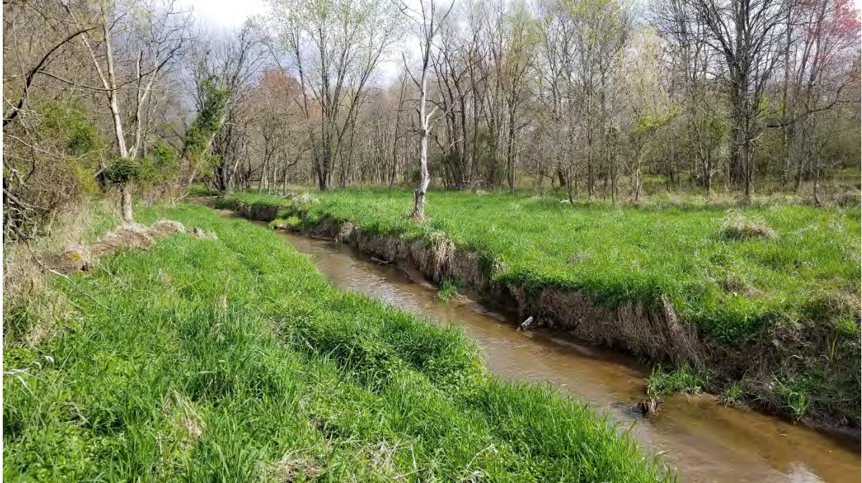
Photo 10: Plumtree Branch is incised with near vertical banks. The banks lack deep rooted vegetation to help stabilize the channel.
