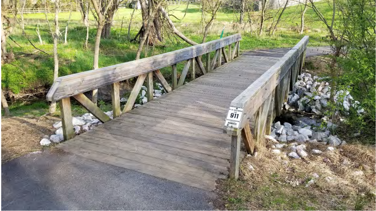
Photo 1: Existing bridge over the unnamed tributary to Plumtree Branch.
