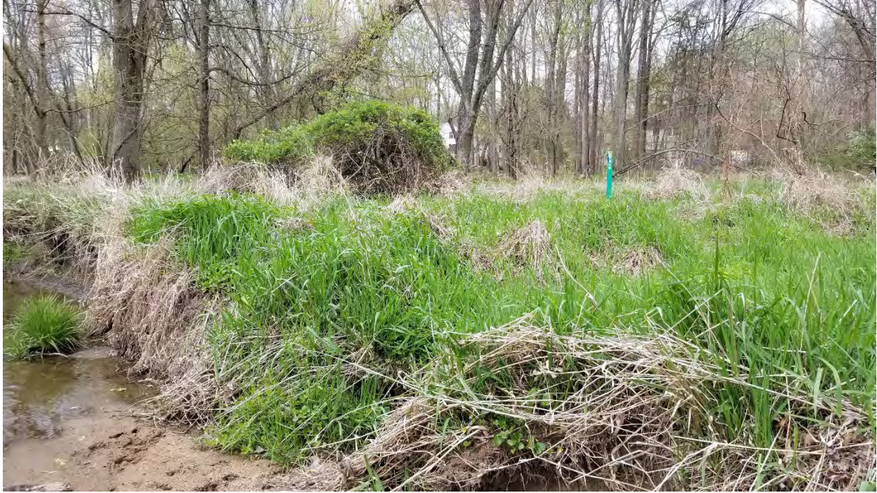
Photo 12: Sewer line near Plumtree Branch. The sewer runs parallel to Plumtree Branch and crosses under the stream at several locations.
